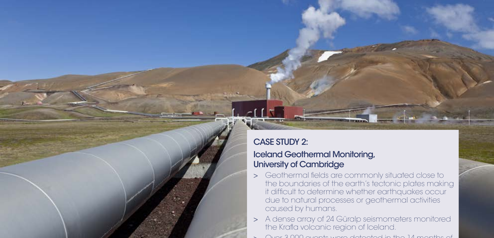
IMAGE 2: KRAFLA GEOTHERMAL POWER PLANT, ICELAND
